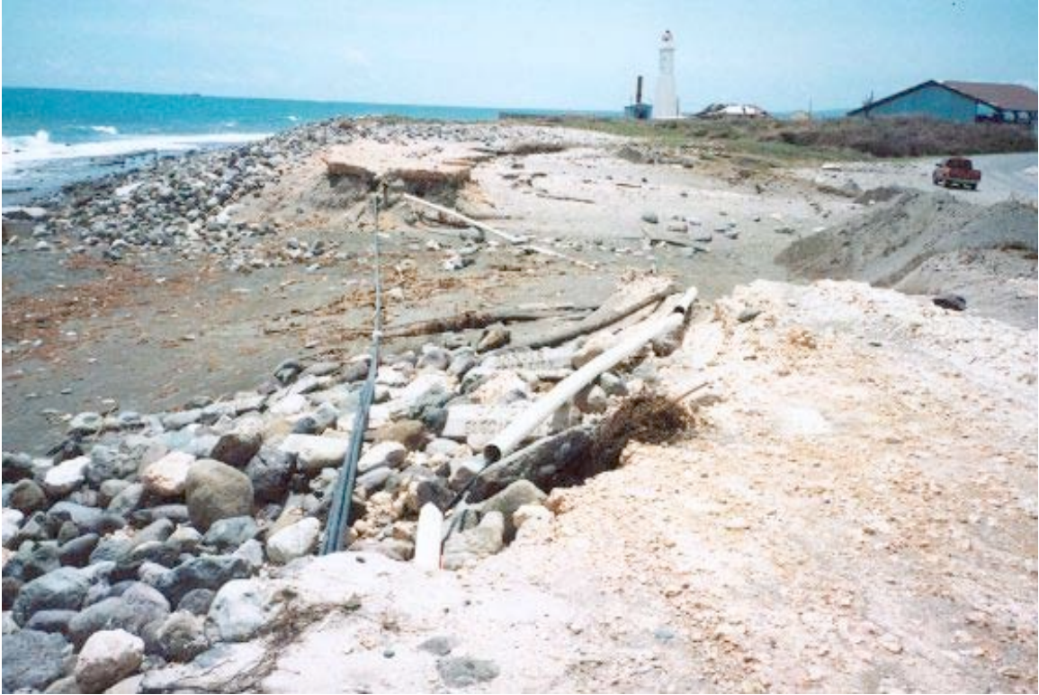
Figure 9: Hurricane Ivan's Disruption of Shoreline at Eastern End of Runway, NMIA
